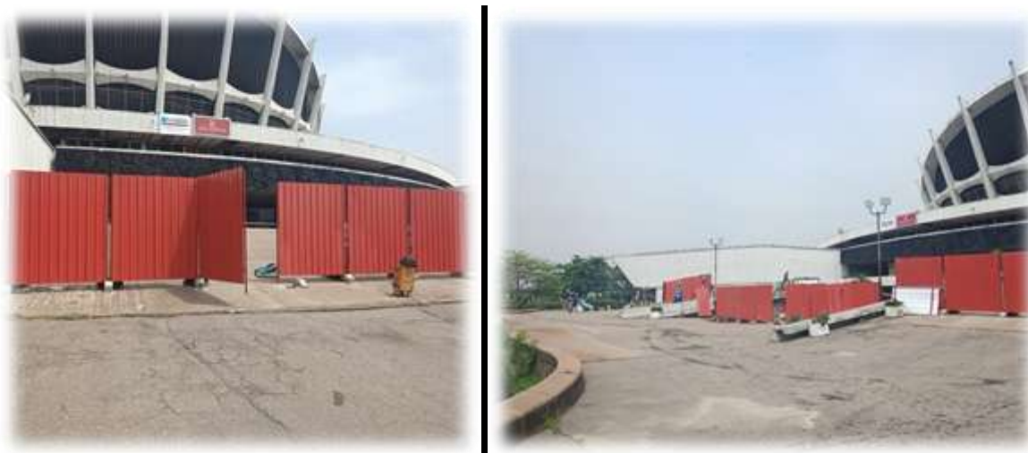
Figure 4 - Hoarded Structure for Rehabilitation (Source: Author's Field Survey, 2021)
