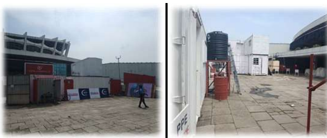
Figure 5 - Pictures Showing Equipments and Containers for Work (Source: Author's Field Survey, 2021)
