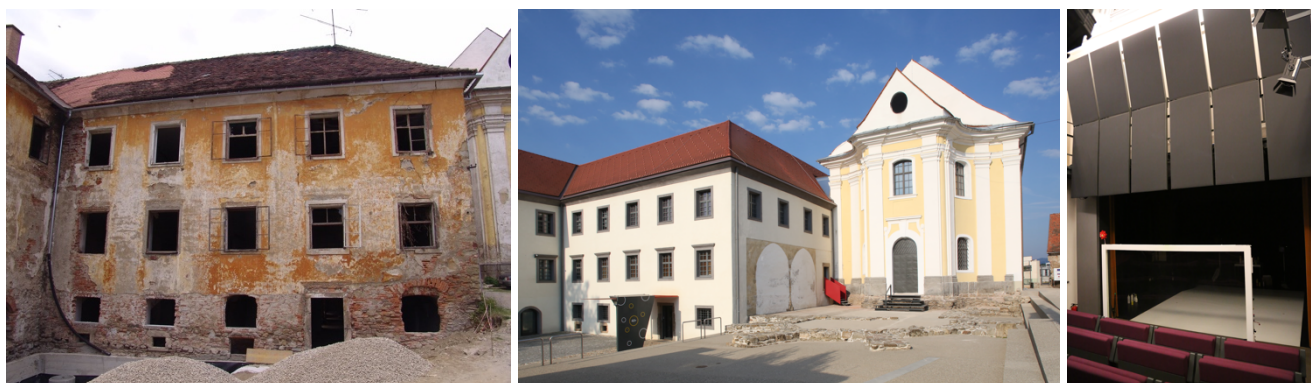
Figure 1: The Minorite complex prior to renovation in 2005 and after renovation (Source: photography by Igor Sapač)
