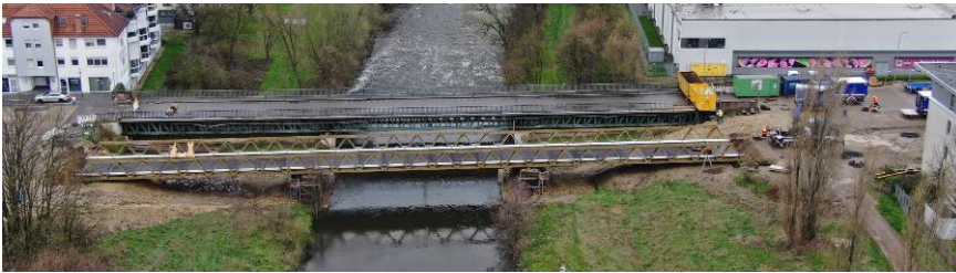
Figure 11: Fully erected temporary bridge
